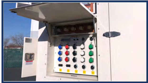
CUSTOMER CONNECTION PANEL
