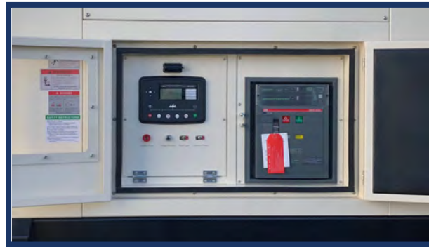
REAR CONTROL PANEL WITH MLCB
