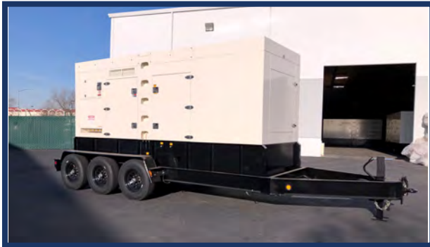
LARGE 600 GALLON CAPACITY FUEL CELL
